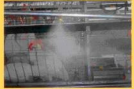
High / low pressure fogger system
